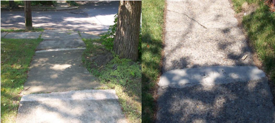
Edge Grinding\* (the light portions of the Sidewalk have been ground down)
